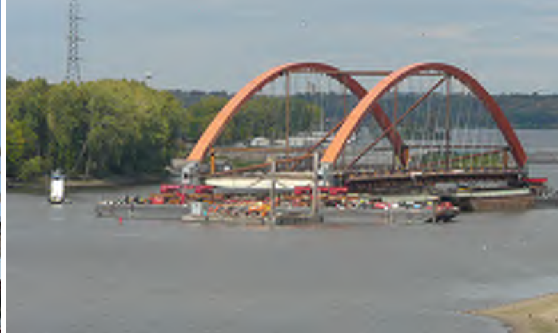
Figure 7: Float-in Construction - Hastings Bridge, MN
