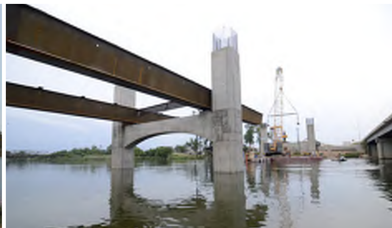
Figure 18: Construction of the Brazos River Bridge Superstructure with Barge Mounted Cranes
