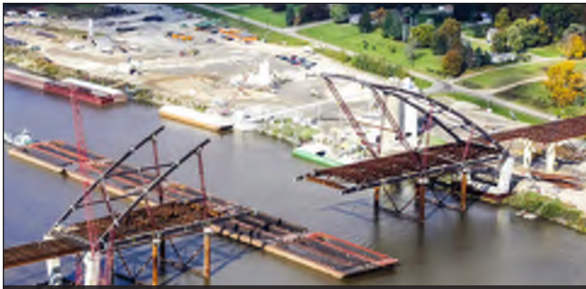
Figure 8: Falsework Construction - Blennerhassett Bridge, WV
