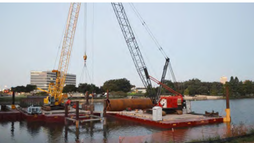
Figure 17: Construction of the Brazos River Bridge Foundations with Barge Mounted Cranes
