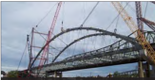
Figure 10: Tieback Tower Steel Erection - Amelia Earhart Bridge, KS
