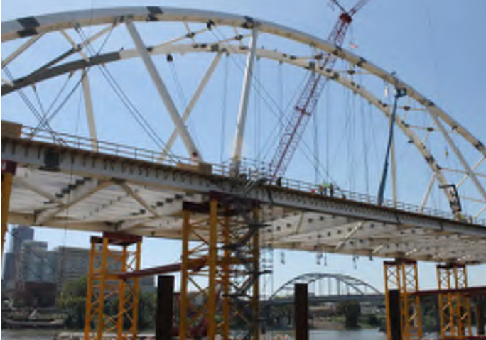
Figure 6: Offsite steel erection - Broadway Bridge, AR
