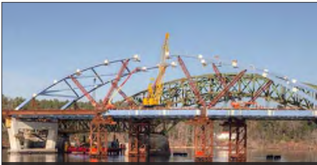
Figure 9: Falsework Construction - Whittier Bridge, MA
